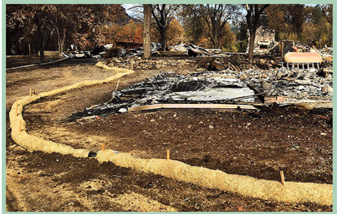
Straw wattles were staged by volunteers trained by the U.S. Fish & Wildlife Service. Photo courtesy of the Friends of Butte Creek.
